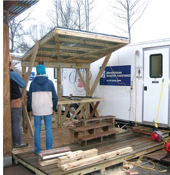
Roof in normal upright position
